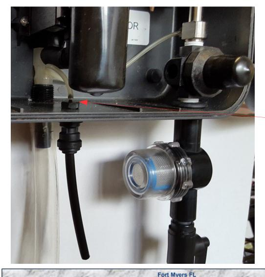
Image to the left shows completed installation of the bypass assembly drains. Image includes an modification to the intake to include plumbing the TEE Strainer directly onto the cabinet, there is a shut off valve (not part of the bypass kit) shown beneath the TEE Strainer.
